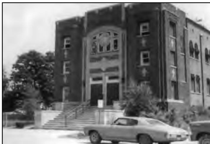
Beth Tephilath Moses dates to 1909 when a group of Jewish residents began worshipping at a home on S. Walnut Street in Mount Clemens. In 1911, Congregation Beth Tephilath Moses was officially founded. This building was opened in 1921 to serve the congregation and is still in use today.
